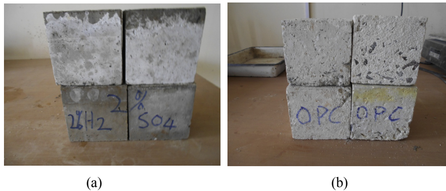
Fig. 1. Visual appearance of four blocks of each (a) GPC3 and (b) M40 concretes after immersing in 2% H 2 SO 4 solution for a period of 90 d.
