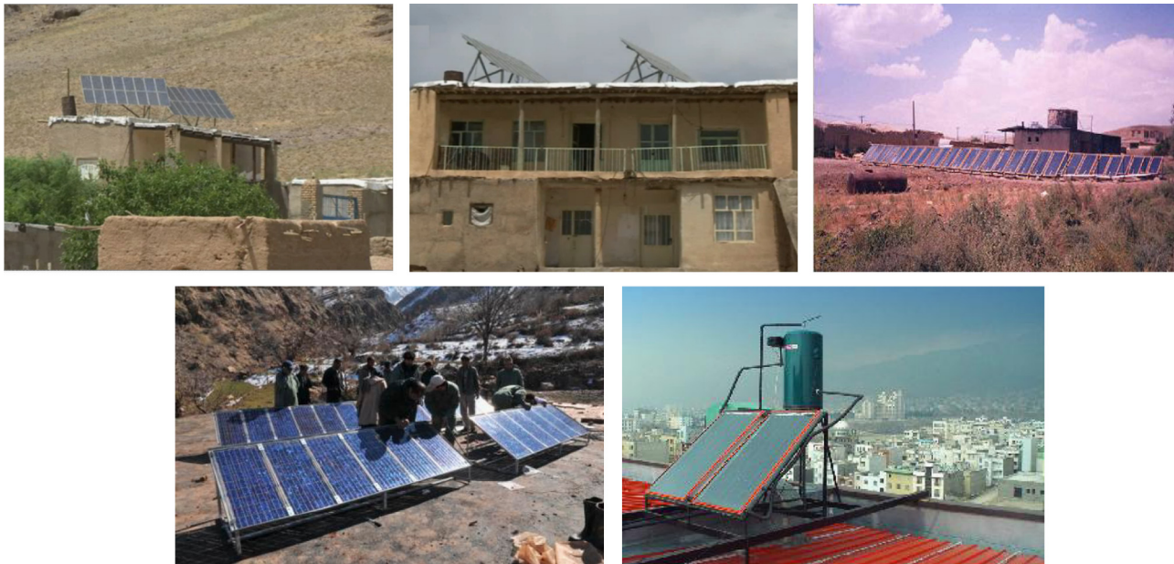
Fig. 16. installing large numbers of solar panels on rooftops around the country—buildings—at over a 1000 new locations specially at rural areas [83,26].
