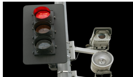
Figure 2: Cameras installed on red light.
