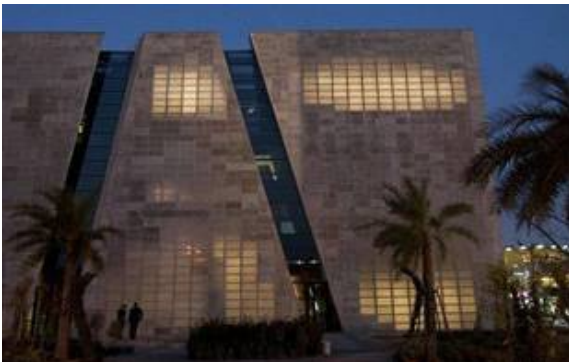
Fig 6. Translucent concrete of Italian Pavilion
