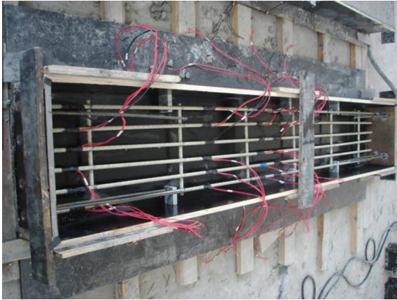
Fig. 4. Reinforcement layout in frame work before casting.
